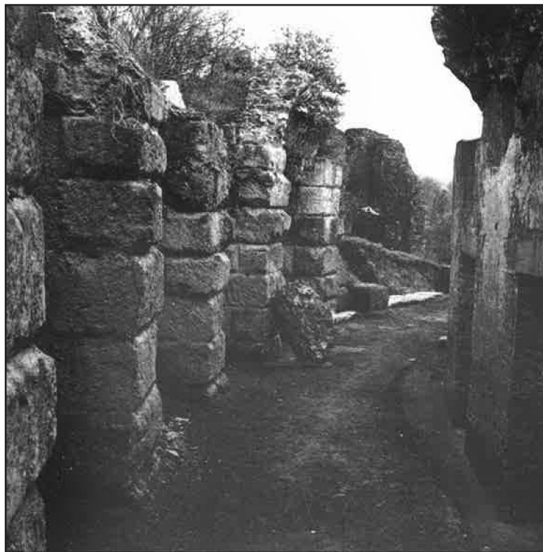
Upper ambulatories: pillars in squared tufa blocks
